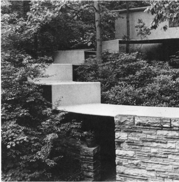
Fig. 16. Continuous structure in reinforced concrete; the folded plane, the circular form with compression on the inner circumference, and minimal uprights (not visible in the photograph) make this a splendid demonstration of cantilevering. Fallingwater, 1939 (Paul Mayén).
